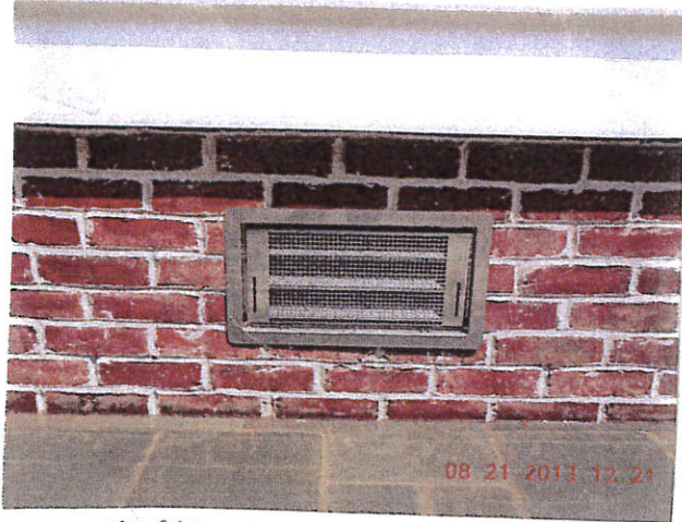
SMART VENT - TYPICAL OF 5 (TOTAL)
