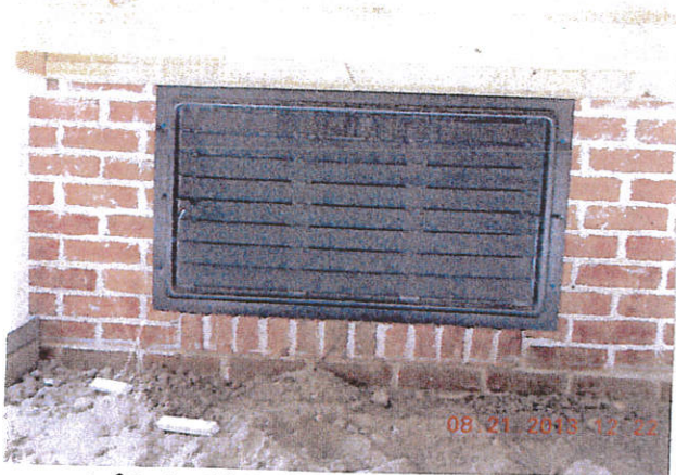
CRAWL SPACE DOOR SYSTEMS VENT TYPICAL OF 2
